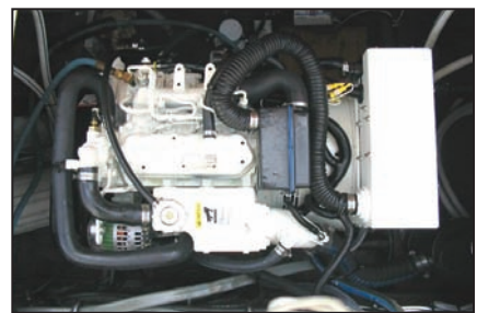
(top) Removing the old, rusty gen-set exposed an inadequate bonding system and resulted in a labor-intensive upgrade. (bottom) New 8kW Kohler fits the hold.
